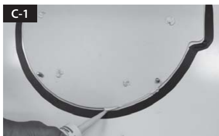
Apply silicone around mounting plate
