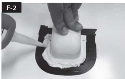
Apply silicone around cable holder
