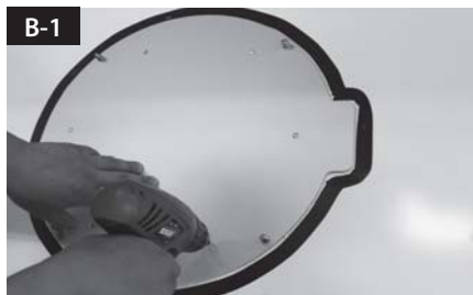
Put back the mounting plate on the silicone applied and make 6holes (2mm) with power drill
