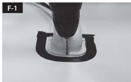
Place cable holder in the tape marked and make 3 of 2mm drill holes
