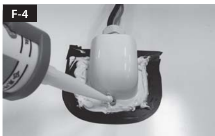
Apply silicone around and on the top of screws
