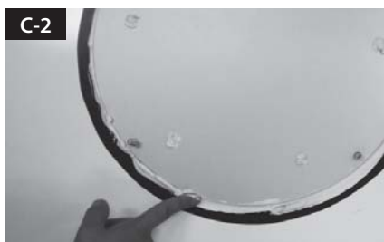
Tidy the area silicone applied
